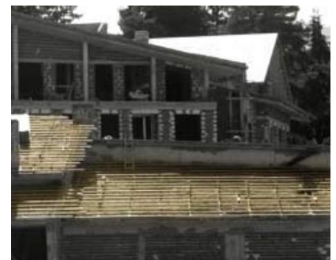
Insulation between roof frame elements with FIBRANgeo R-050
