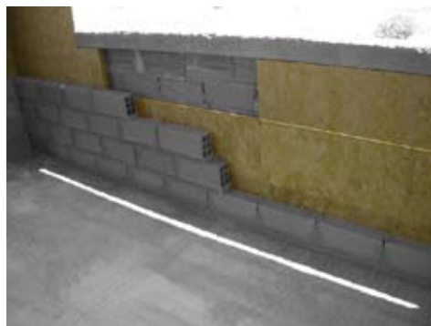
Masonry cavity wall insulation with FIBRANgeo B-040
