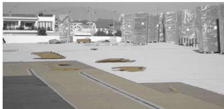
Steel roof with double layer of insulation with FIBRANgeo BP 50 + BP 70
