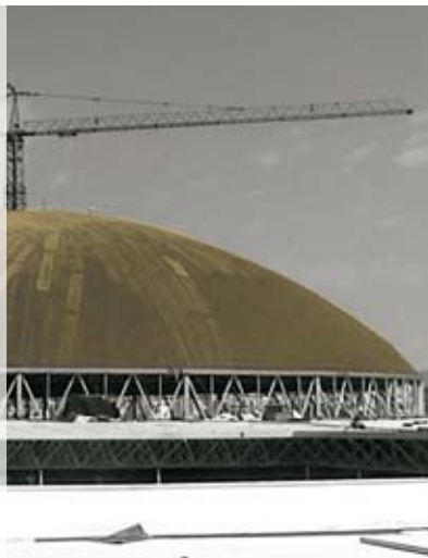
Steel deck with double layer of insulation with FIBRANgeo BP70 + BP 40
