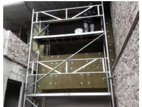
ETICS system with FIBRANgeo BP-021
