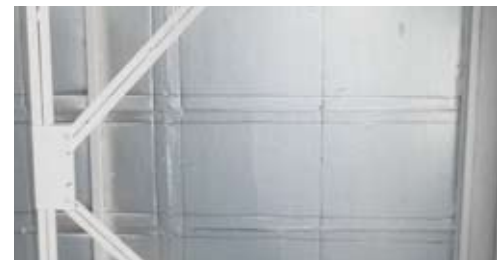
Exposed internal insulation of metal roof cladding with FIBRANgeo B-570-AX
