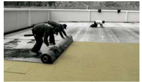
Steel deck with waterproofing membrane with double layer of FIBRANgeo BP 40
